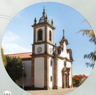
146 Parish Church of Sambade Sambade
