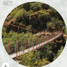
Mineiros Bridge Argozelo
